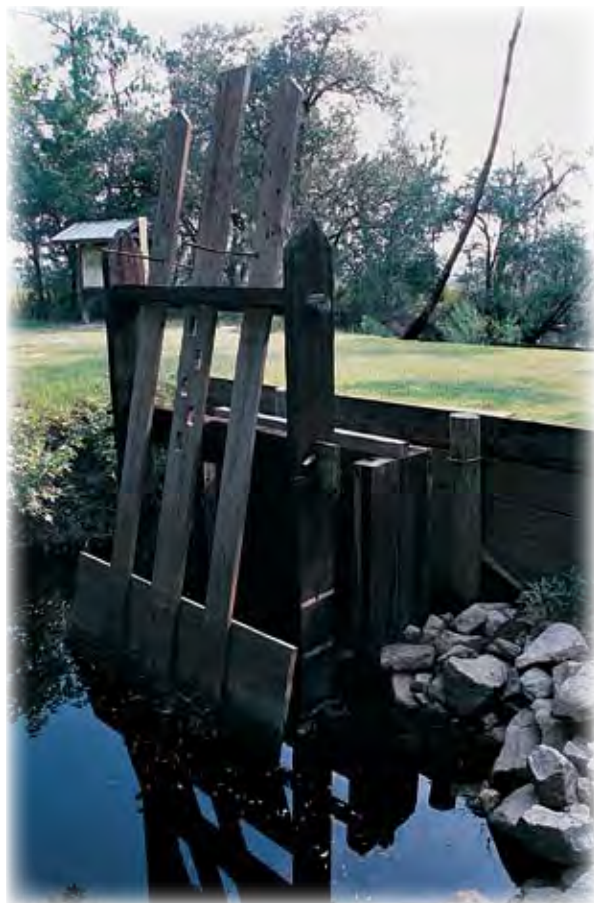
Rice trunks like the one pictured here are an important tool in the management of freshwater impoundments. They are used to control waterflow between tidal rivers and impoundment systems.
