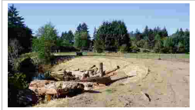
Clallam River Bank Stabilization at Sadilek Farm
